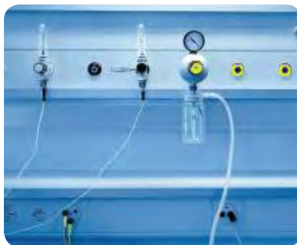
Complete bedhead panels installed at hospital
